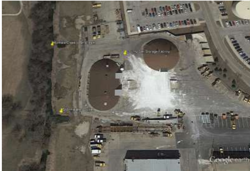
Plate 7. Google Earth image of the DuPage County salt storage facility on Winfield Creek suspected of contributing to chloride violations 0.6 miles downstream in 2009 and 2012. An apparent stormwater outlet to Winfield Creek is noted immediately west (to the left) of the facility.
