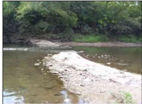
Plate 2. Remnants of the McDowell Grove dam used to form a riffle after its removal in 2008. The riffle and former structures remain in place.
