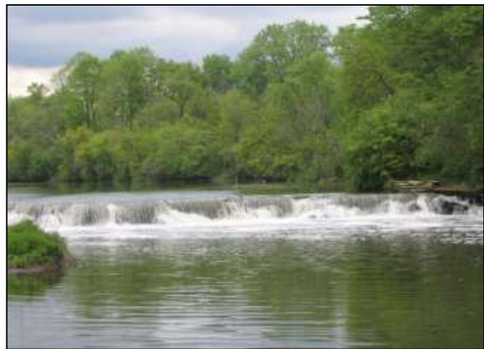
Plate 1. The former Warrenville Grove Dam, looking upstream. The dam was removed in 2011.
