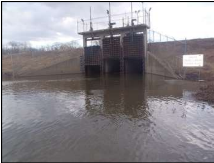
Plate 5. Upstream view of the Fawell Dam.
