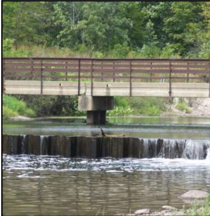
Plate 3. Temporary cofferdam constructed upstream from the former McDowell Grove Dam in 2008. The cofferdam was removed in the fall of 2012, immediately after the 2012 survey.
