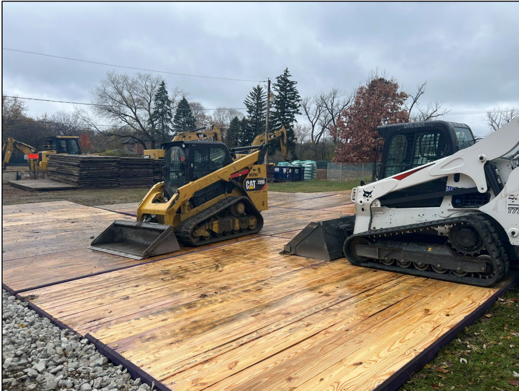
Plate 2. Photograph of the construction staging area at Fullersburg Woods (November 2023).
