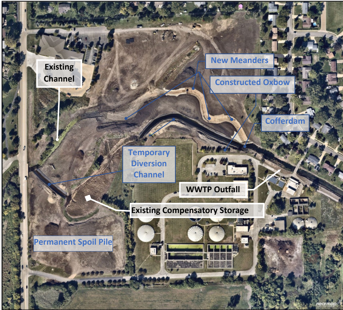
Plate 19. Aerial photograph of Klein Creek Streambank Stabilization Project (October 2022) By mid-October 2022 approximately \frac{2}{3} of the new channel had been excavated, with about \frac{1}{2} having also been filled with the new streambed material. Construction proceeded from upstream to downstream (east-to-west; right-to-left). The temporary diversion channel is to the south and partially cuts through an existing compensatory storage basin to save costs.
