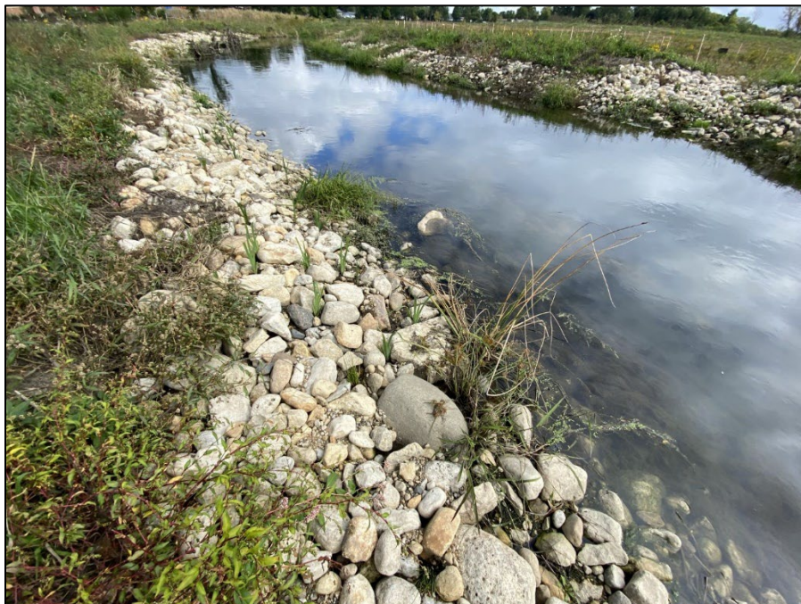
Plate 32. Looking downstream at the recently planted plugs within the vegetated rock toe.
