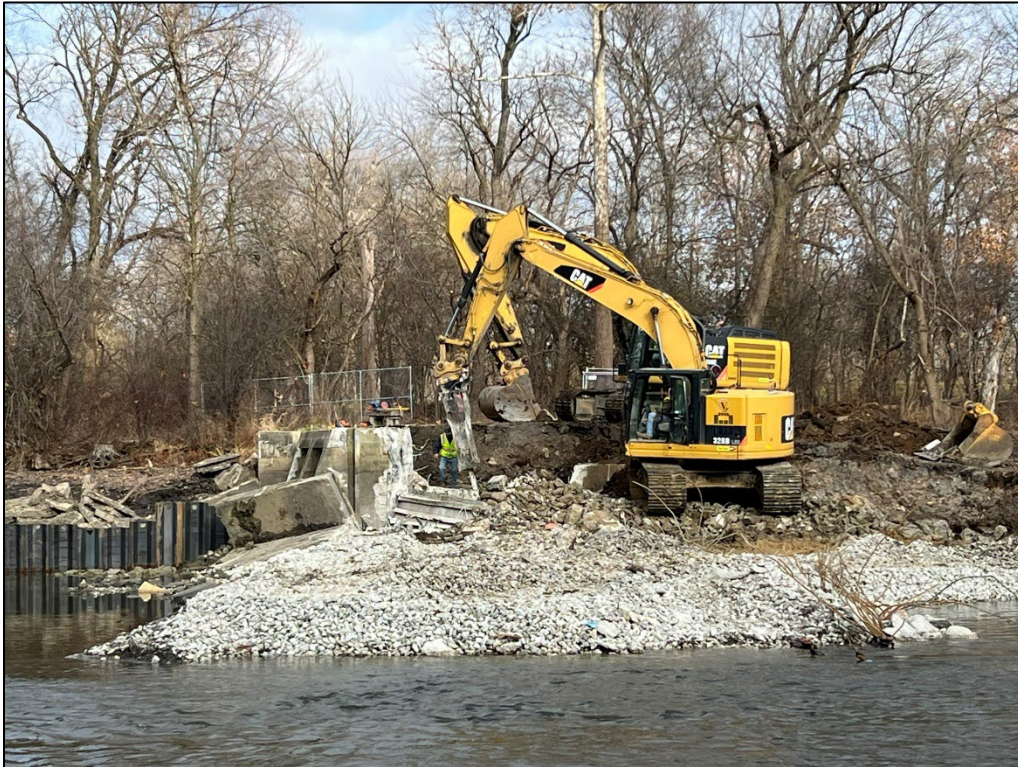
Plate 10. Photograph of the demolition of the dewatering structure (December 11, 2023).
