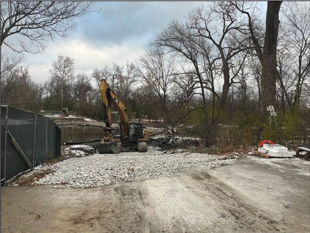
Plate 4. Photograph of the installation of the causeway upstream of the dam (November 29, 2023).
