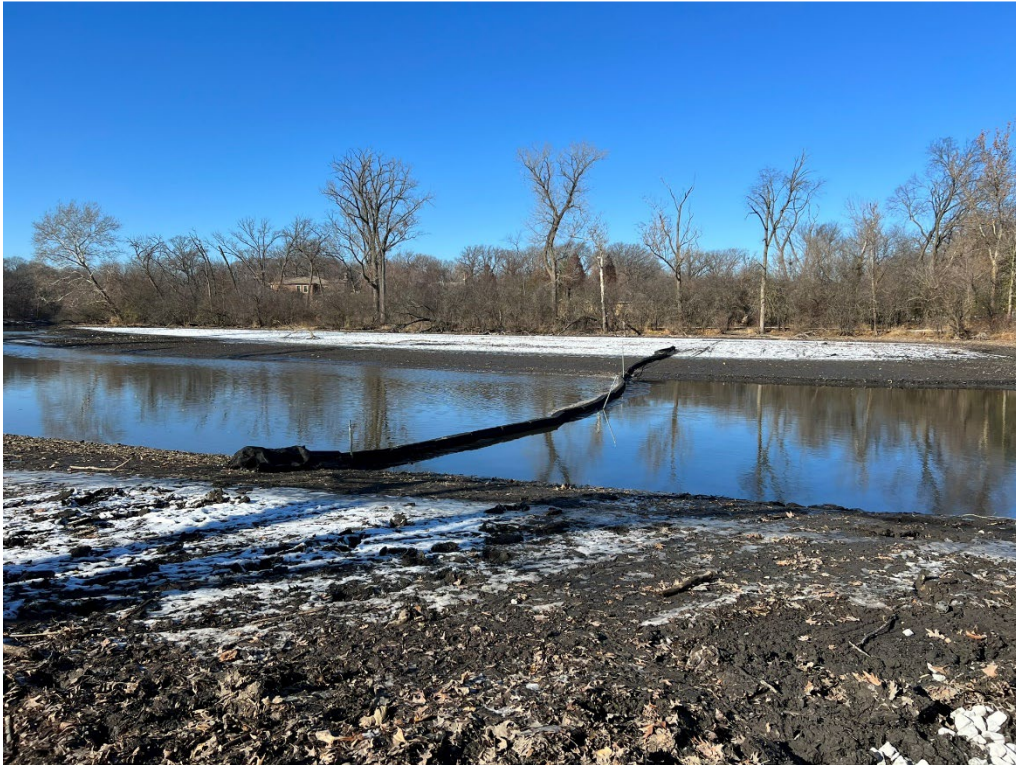
Plate 5. Photograph of one of the silt curtains utilized in the instream work (November 27, 2023).
