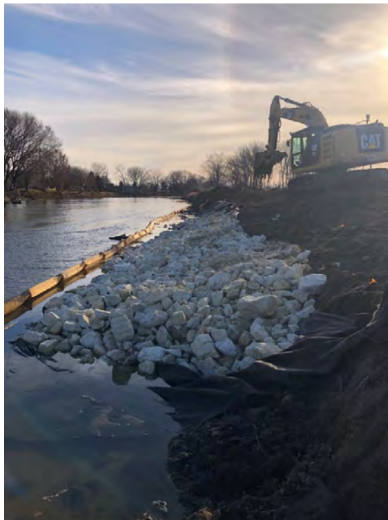
Plate 19. Photograph of the boulder toe installed on the west bank of the DuPage River (Winter 2025)
