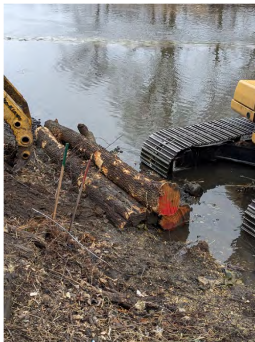
Plate 25. Photograph of a brush box being installed on the east side of the Lower DuPage River (Winter 2025)
