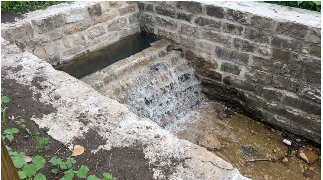
Plate 14. Photograph of the cascade in the re-design Graue Mill raceway
