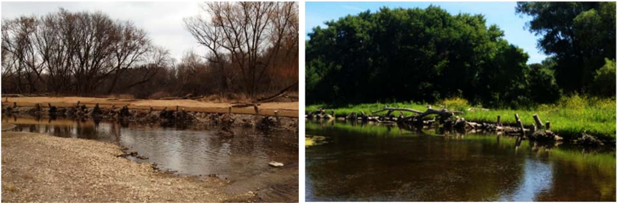
Figure 12. Large wood crib structures, Sheboygan River, Wisconsin. During (left) and two years after construction (right).
