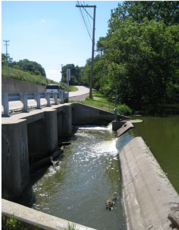
Former Churchill Woods dam (E. Branch RM 18.6 at Crescent Rd. (Note: dam wall removed in February 2011).
